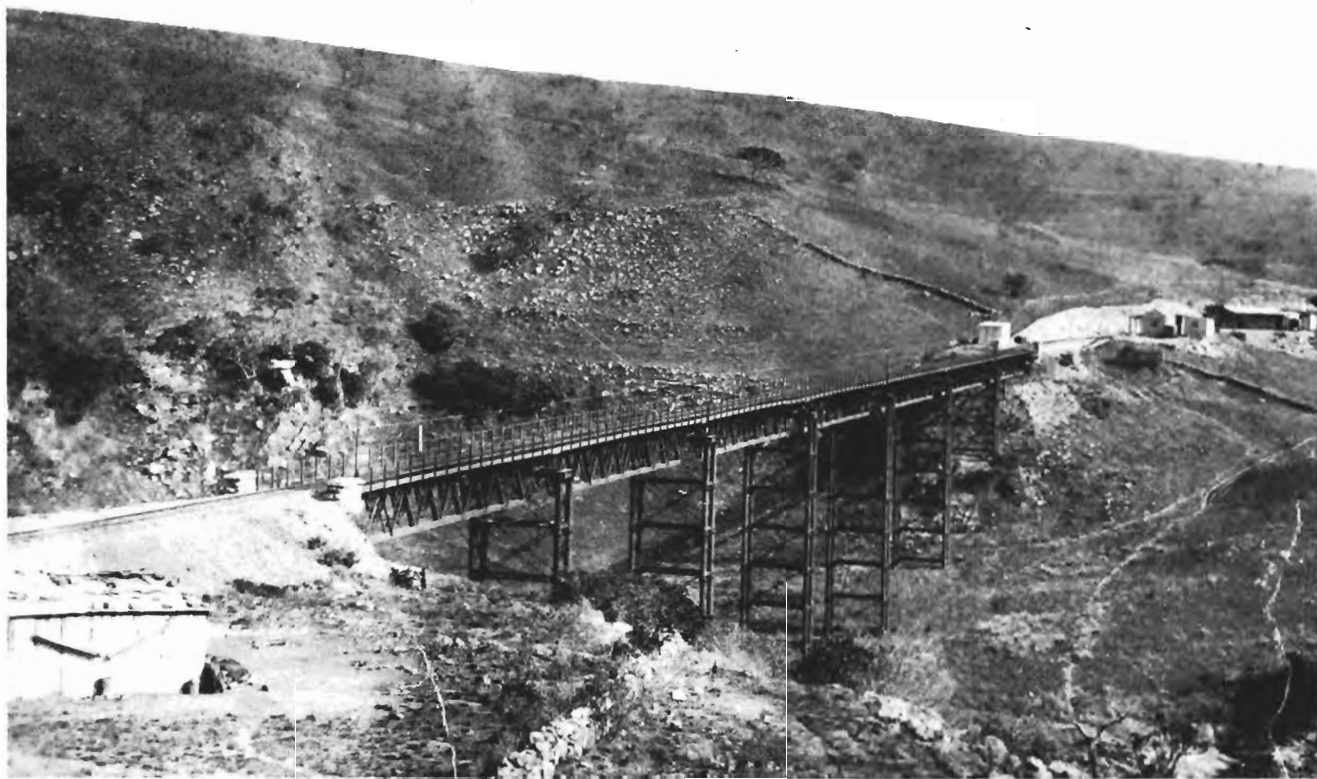
The Inchanga Viaduct (567 ft.), completed in March 1880
