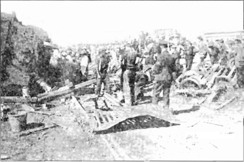
*CLEARING THE WRECKAGE. On the right is one of the bogies of the tram-car wrenched from its fittings. In the foreground is the cow-catcher of the locomotive which struck the tram and was torn off. The rear tender of the engine, lying on its side, is shown at the side of the picture.*
