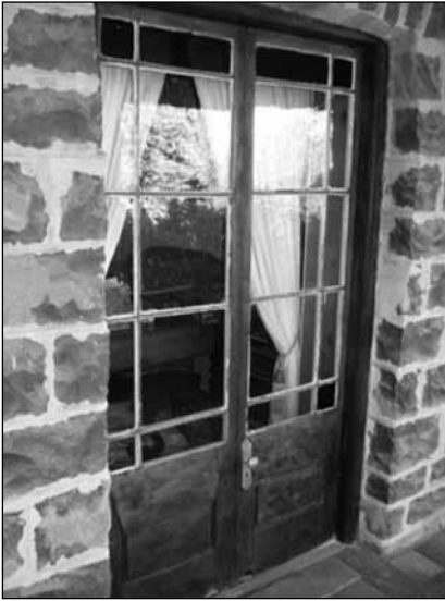
The 18-inch ironstone walls of the main building date back over a century
